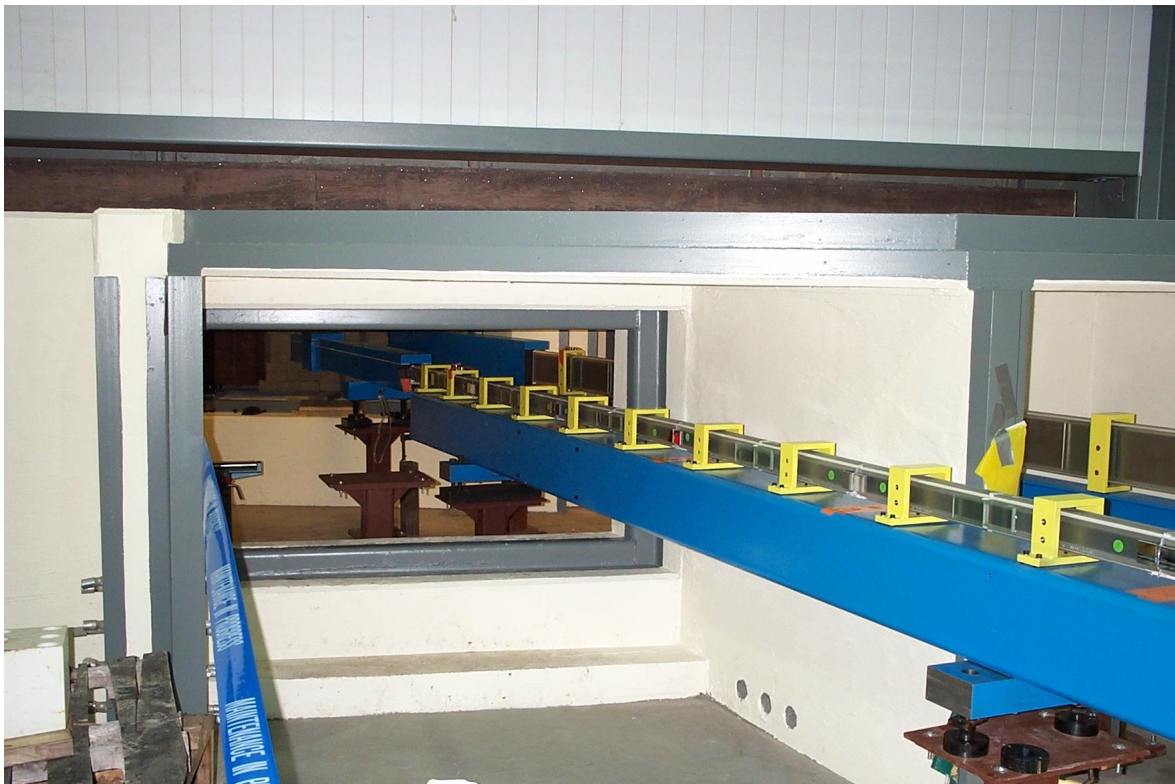
Figure 6: Installed CG-1 and CG-2 Guides at the Entrance to the Guidehall
