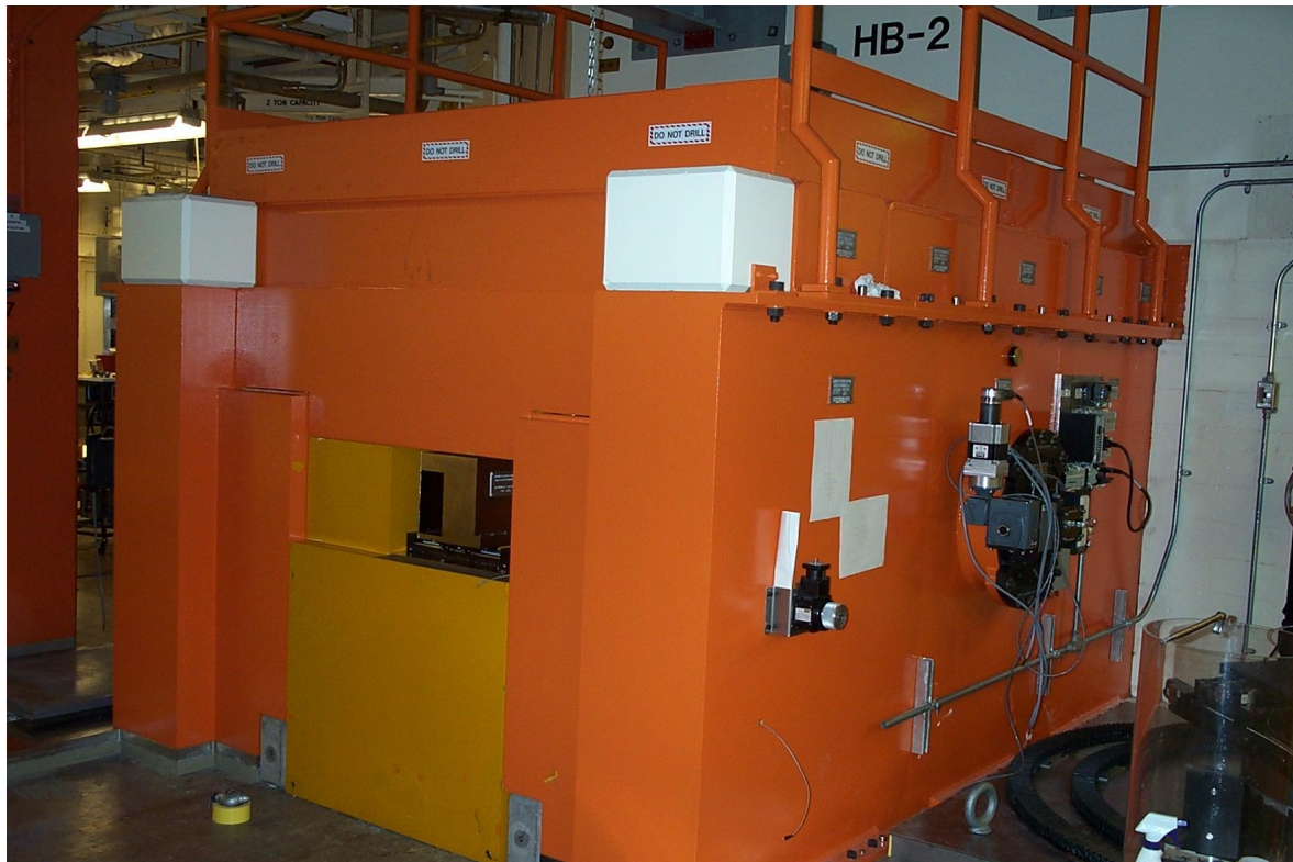
Figure 3: West and South Faces of the HB-2 Shield Tunnel
